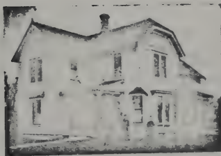
RESIDENCE OF FULTON STREAM, SPAULDING, IOWA.
